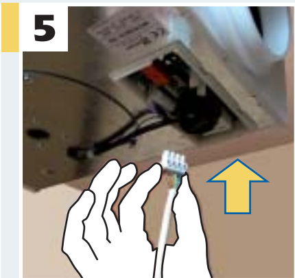
5 Fix the connected terminal into the integral junction box
